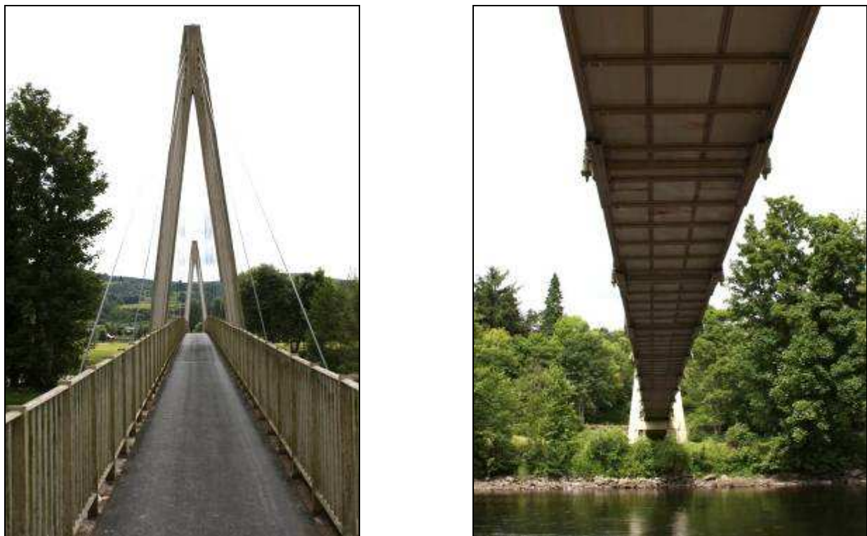
Figure 4. Aberfeldy footbridge from above and below the bridge deck (June 2008)
