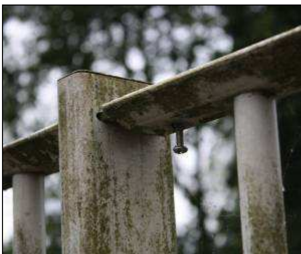
(a) Screw repair (June 2008)
