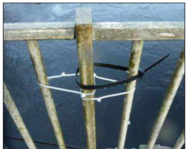
(b) Zip tie repair (December 2011)
