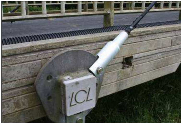
Figure 7. Anchorage of a cable to the bridge deck (June 2008).
