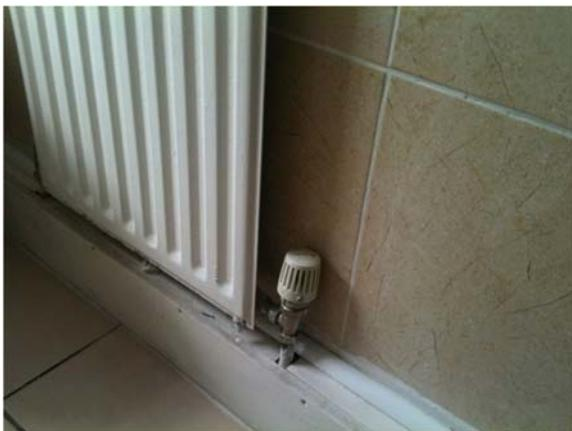
**Fig. 4** Radiators 'locked in' by boxed away pipes
