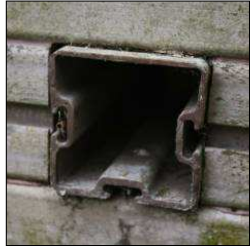
(b) The sealed end of a transverse beam
