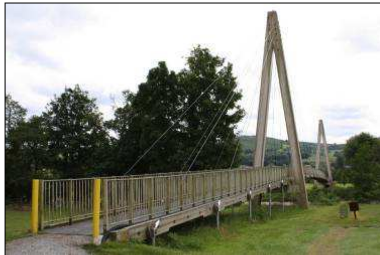
Figure 2. Aberfeldy footbridge from the north (June 2008).
