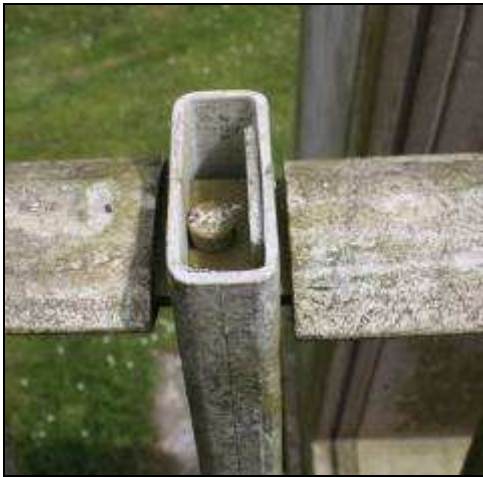
Figure 12. Details of the connection between the top handrail and parapet post (June 2008).
