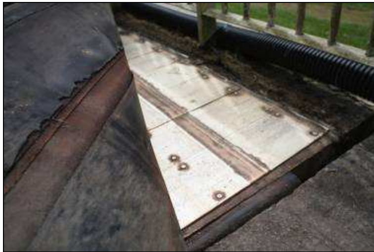
Figure 5. GFRP plates retrofitted to strengthen the bridge deck (June 2008)
