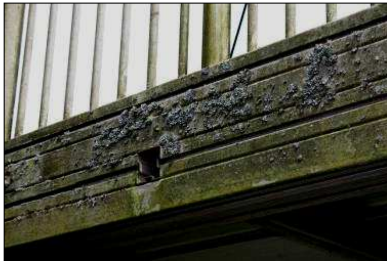
Figure 10. Greening of the bridge deck (June 2008).
