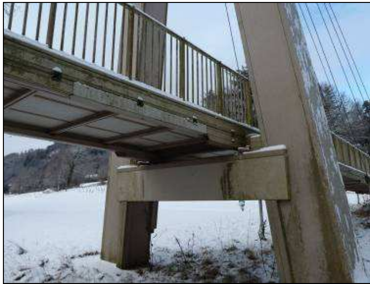
Figure 16. Impact protection applied beneath the deck (December 2010).
