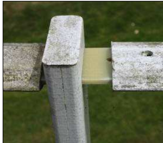
Figure 12. Details of the connection between the top handrail and parapet post (June 2008).
