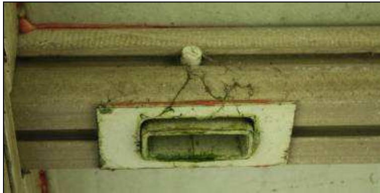
Figure 11. Connection of the parapet post beneath the bridge deck (June 2008).
