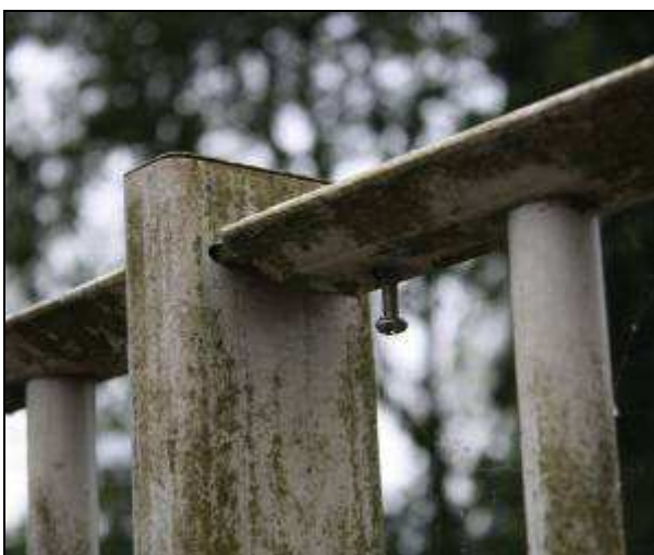
(a) Screw repair (June 2008)
