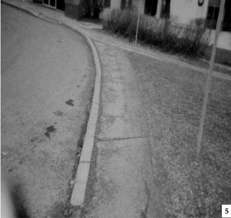
The sidewalk the woman must use to return home is sloped and in poor repair.
